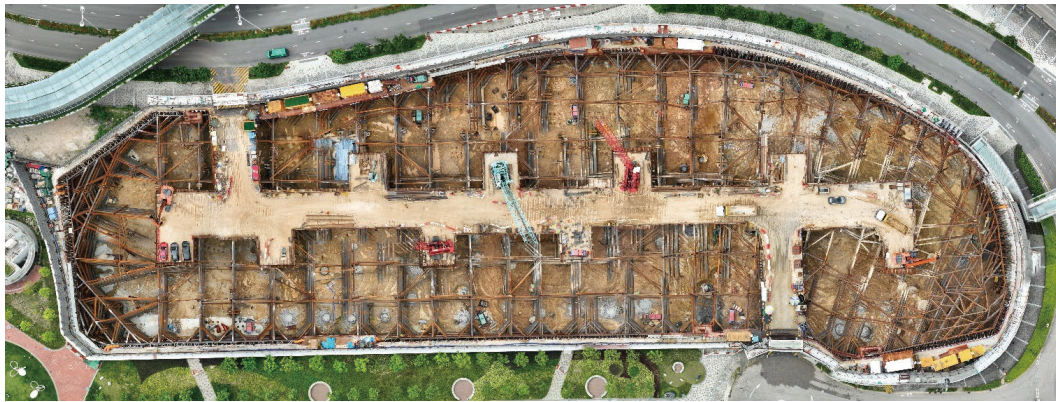
Temporary Steel Working Platform
